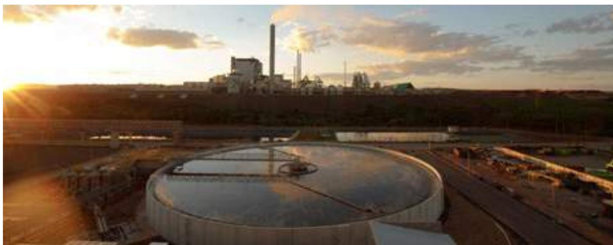
Sludge drying: installation of a drying plant for sludge from effluent treatment, currently in progress at the Puma Unit. In addition to reducing the amount of biological and tertiary sludge to be treated, this presents the opportunity to use the dry sludge as fuel for burning biomass in the biomass boiler.
