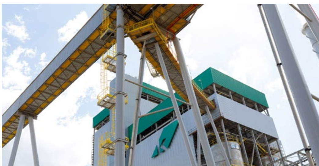
Biomass boiler at the Puma Unit. Photo: Klabin.
