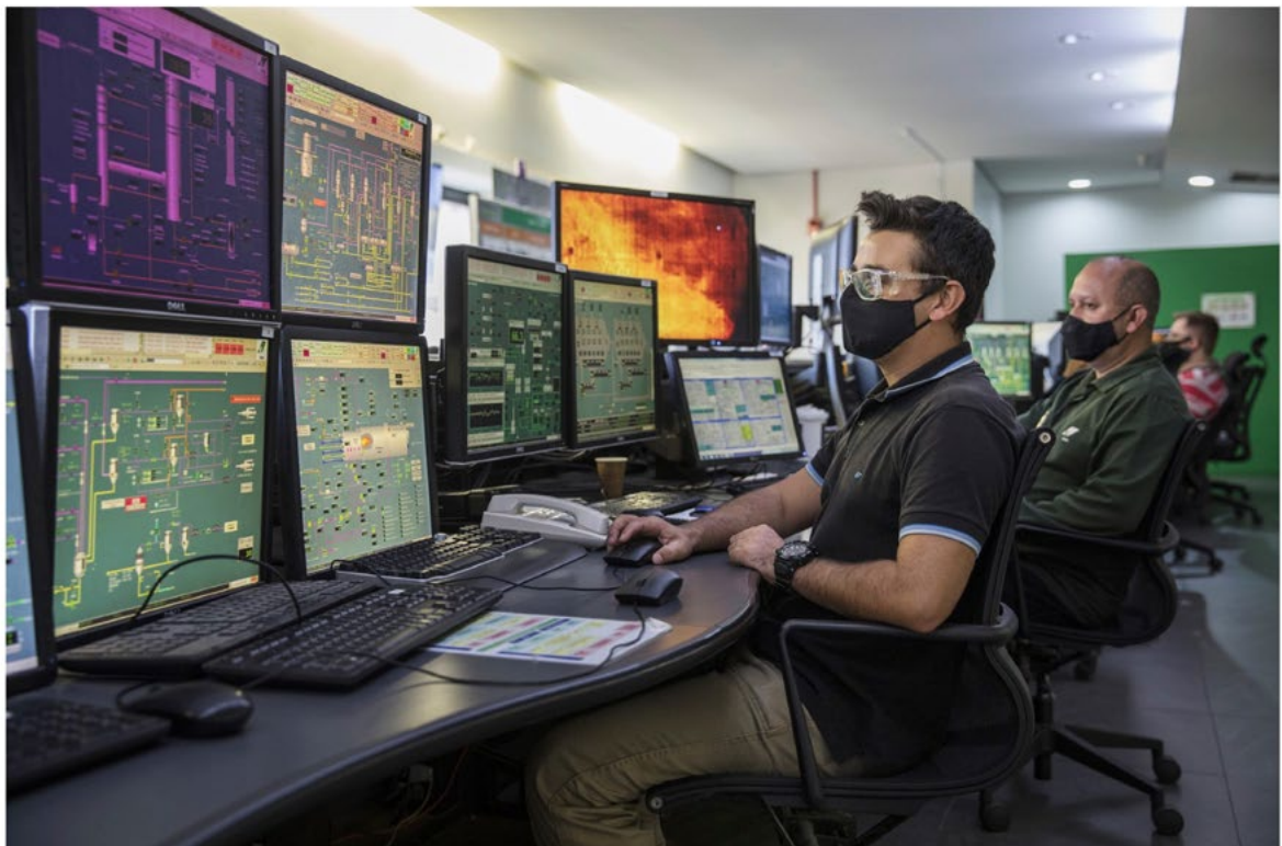
Control Room of the Monte Alegre Factory in Telemaco Borba (PR). Photo: Eduardo Knapp / Eduardo Knapp.
