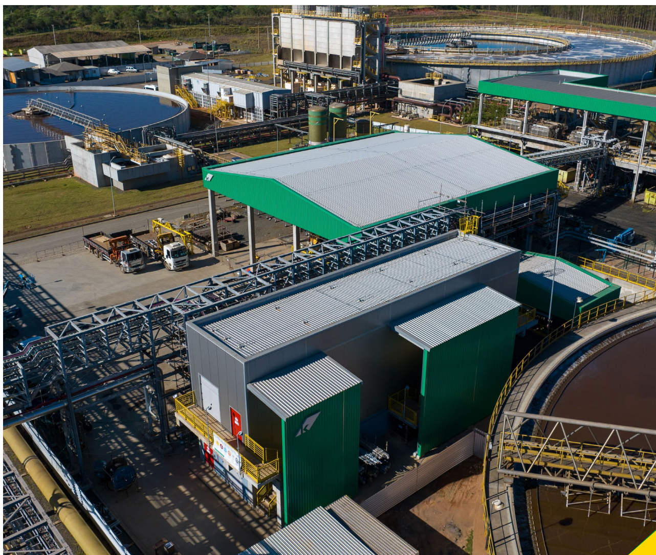
Sludge drying plant in Ortigueira (Paraná)
